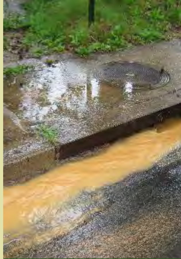
SEDIMENT & POLLUTANT LADEN RUNOFF FLOWS INTO STORM SEWER SYSTEMS.
