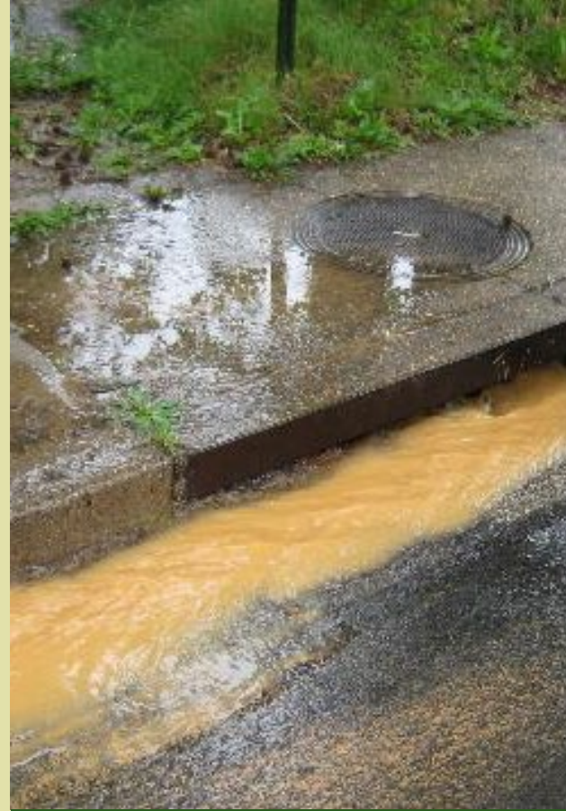
POLLUTANT LADEN RUNOFF FLOWS INTO STORM SEWER SYSTEMS.
